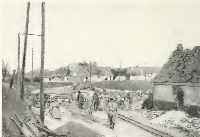
BARRICADE AT NEUVILLE-SAINT-VAAST, IN MAY 1915.
