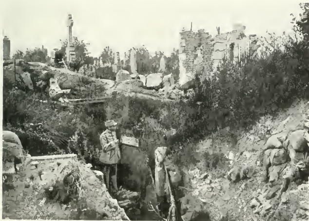
TRENCHES IN THE CEMETERY.
