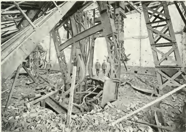
THE ENTRANCE TO COAL PIT NO. 2, AT DOURGES. DESTROYED BY THE GERMANS. The girder-work was dynamited.
