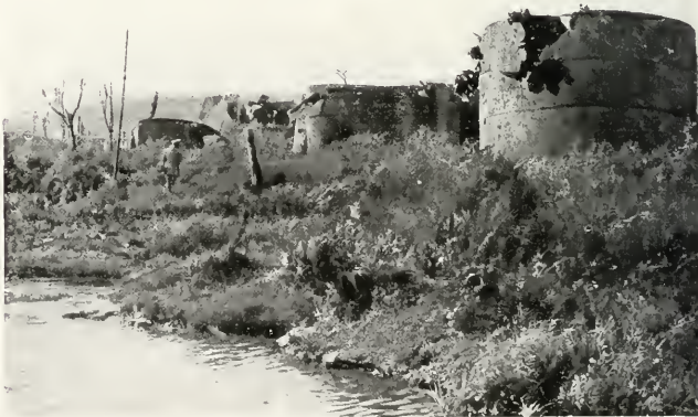
THE RUINED SUGAR REFINERY AT SOUCHEZ.
