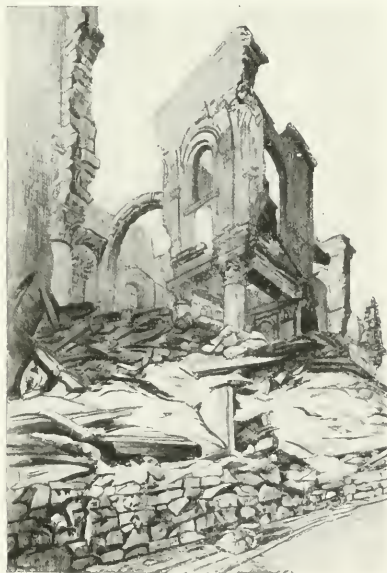
THE COLLAPSE OF THE NORTH TRANSEPT. Drawing by A. Ventre, chief architect to the Historical Monuments Department.
