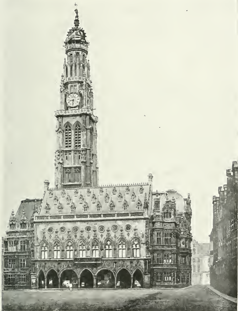
THE HÔTEL DE VILLE AND BELFRY BEFORE THE WAR. The Façade in the Petite Place. Compare with photo, p. 38.
