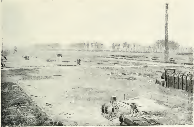
DESTRUCTION OF THE ARBEL WORKS.
