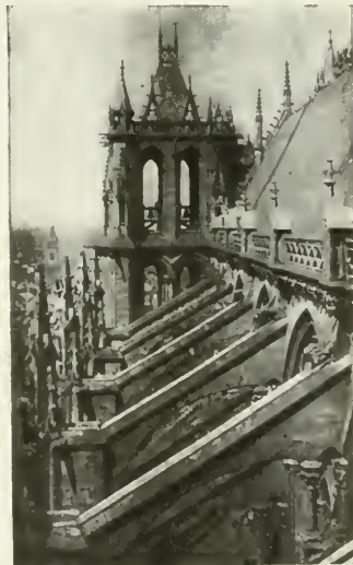
FLYING BUTTRESSES OF NAVE WITH TWO SUPERPOSED ARCHES (Cliché LL)
