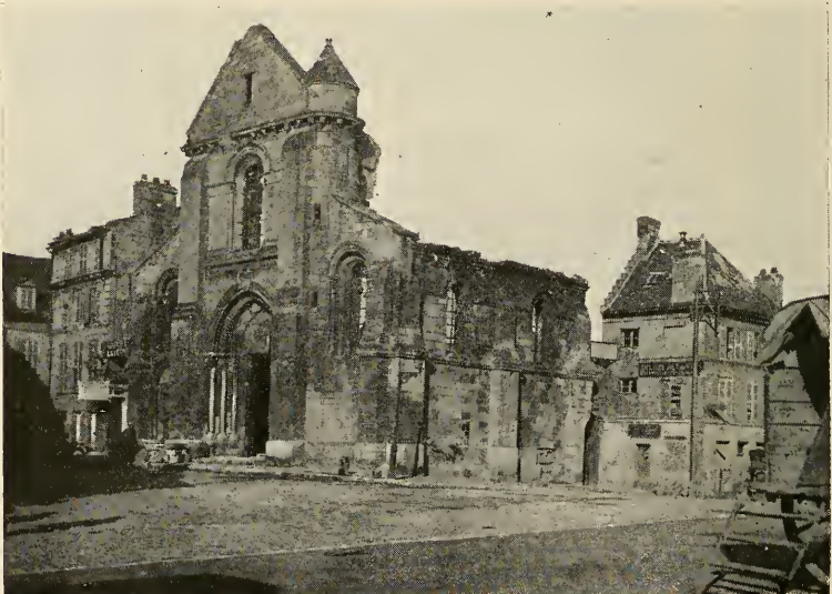
CHURCH OF SAINT PIERRE- AU-PARVIS. November, 1918.
