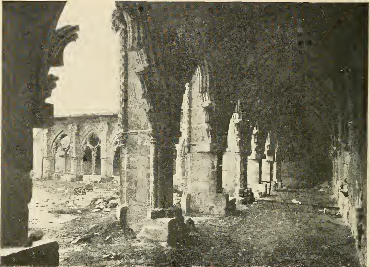
WESTERN GALLERY OF THE CLOISTER. Seen from Doorway. Nov. 1918.
