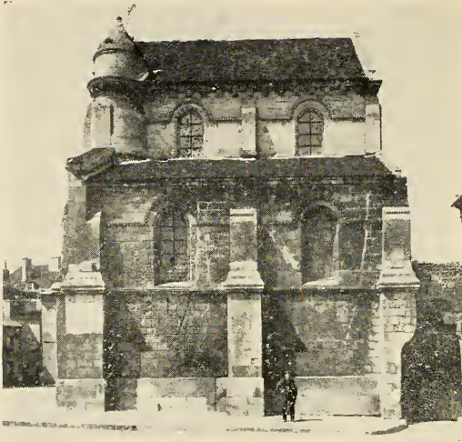
CHURCH OF SAINT PIERRE- AU-PARVIS. South facade before the War.
