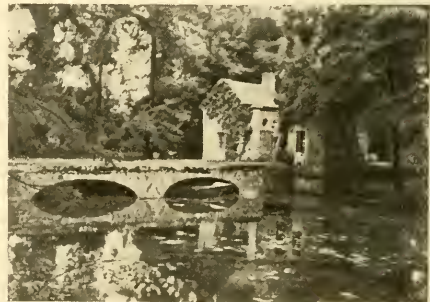
Bridge over the Castle Moat
