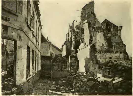
Ruins at the Corner of the Rue du Temple
