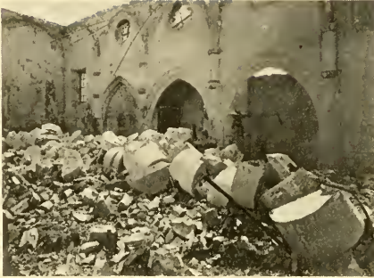
Nave of Huiron Church
