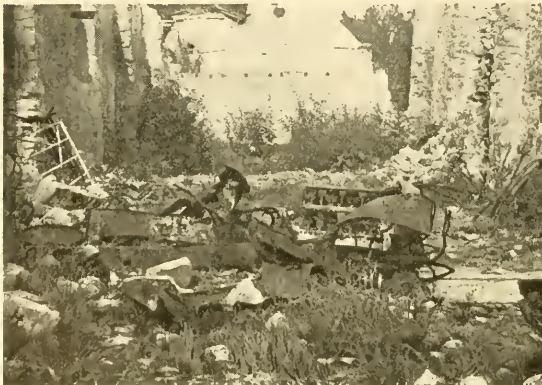
Debris of the Castle Motor Car
