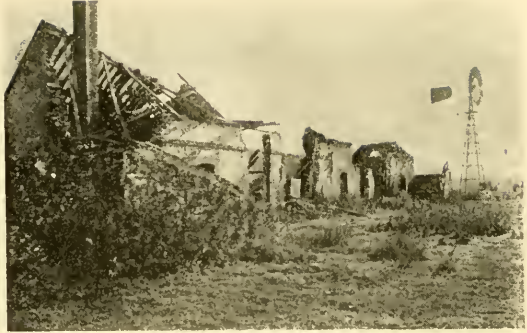
Windmill Water Pump at La Villeneuve
