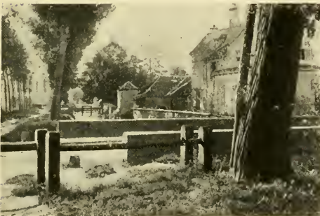
Bridge over an Arm of the Morin
