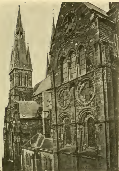
Porch and South Transept of Nôtre-Dame
