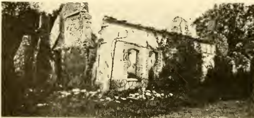
Burned Houses in Champguyon
