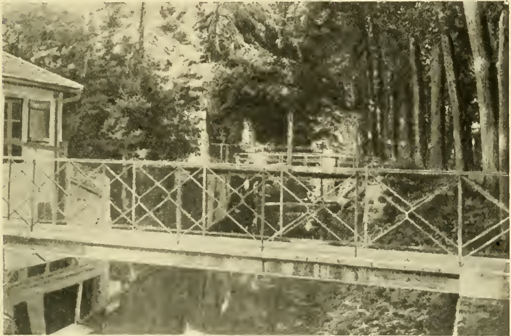
Foot Bridge over an Arm of the Morin
