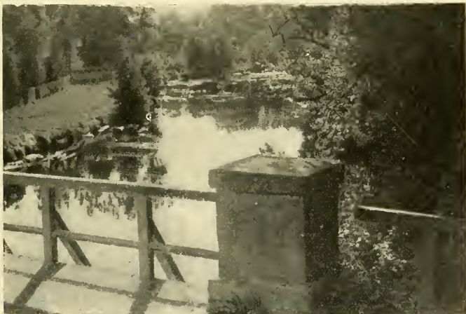
Bridge over the Morin
