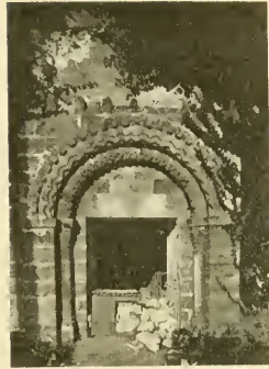
Doorway of Favresse Church
