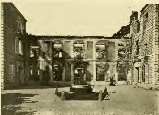
Burned Building, 17 Faubourg St. Martin
