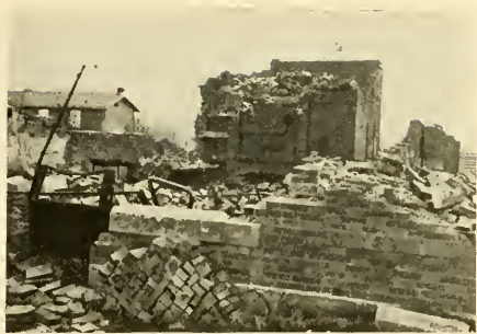
Houses Destroyed in Huiron
