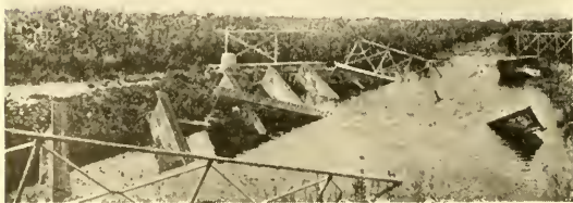
Destroyed Bridge over the Morin
