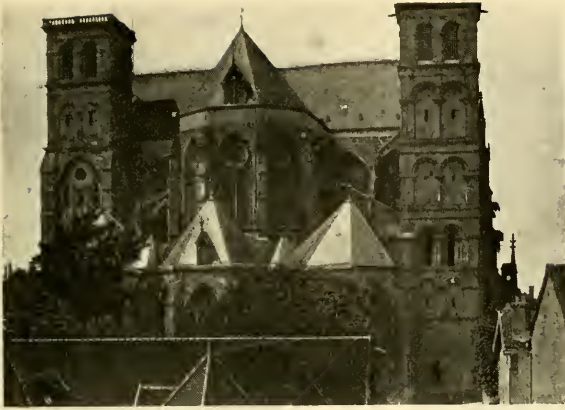
Apse and Transept of the Cathedral
