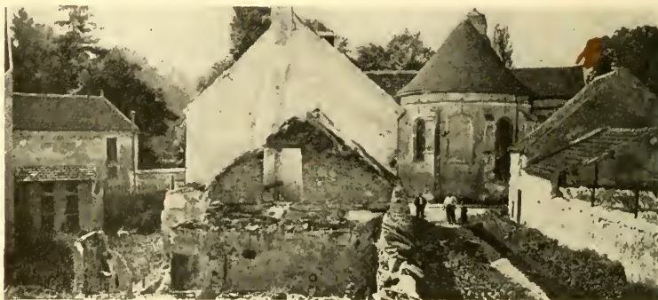
Burned Houses at Chauconin
