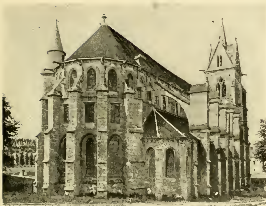
The Church seen from the Road
