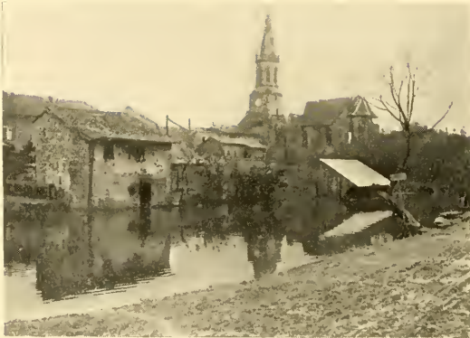
View of Bauzée
