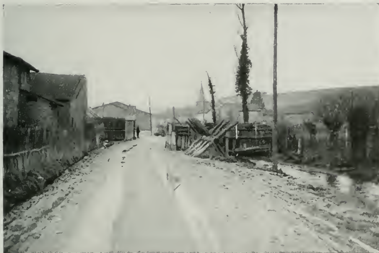
DEFENCE WORKS IN VAUX VILLAGE (JANUARY 14TH 1916).
