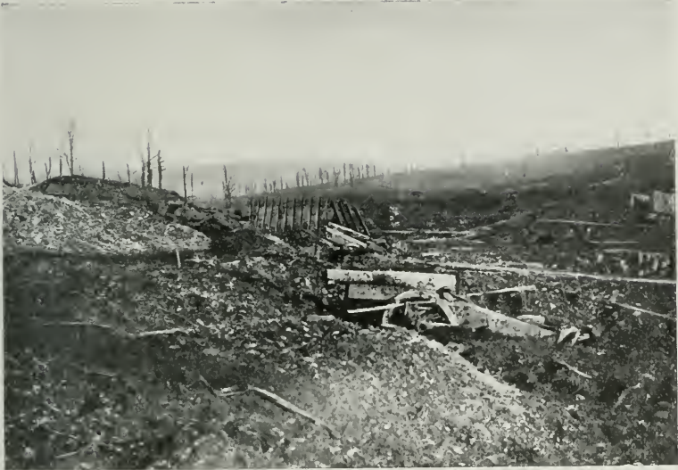
FONTAINES RAVINE IN FEBRUARY 1917. — A demolished French battery.
