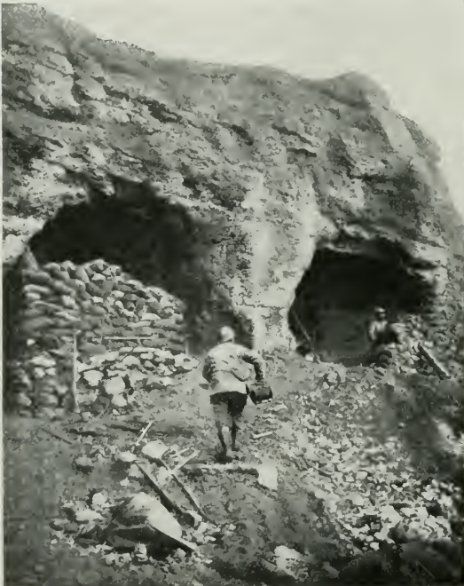
CASEMATES OF VAUX FORT IN NOVEMBER 1916. A signaler reaches the fort.
