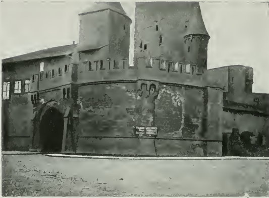
THE PORTE DES ALLEMANDS. View taken from the Quai des Allemands.
