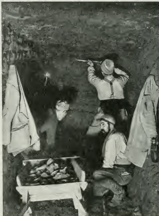
SAPPERS EXCA- VATING A MINE GALLERY.
