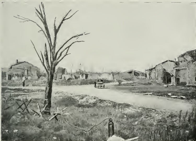
THE RUINS OF MARRE. After passing the church, the car turns right, towards Cumières. On the left, the road to Bourrus woods is impassable.
