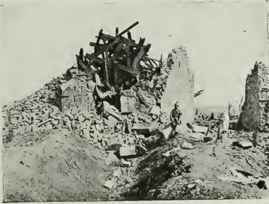
BRAS CHURCH WITH THE RUINS OF THE STEEPLE (APRIL 1917).
