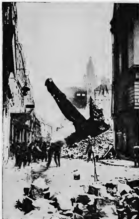
After the bombardment : A Falling House in the Rue de Paris.
