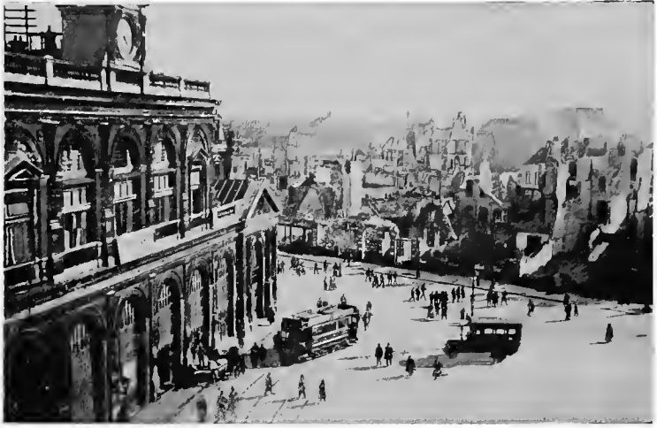
THE STATION AND RUE DE TOURNAI (see p. 15).
