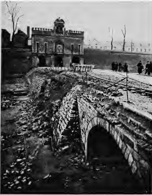
As in the case of the Tournai Gate (p. 34), the retreating Germans blew up the bridge over the moat, seen on p. 57 (before) and above (after) the explosion. A temporary road replaces the bridge.
