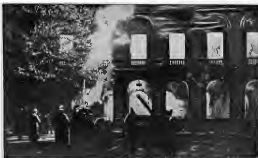
THE HOTEL- DE-VILLE BURNING on the night of April 24 1916.
