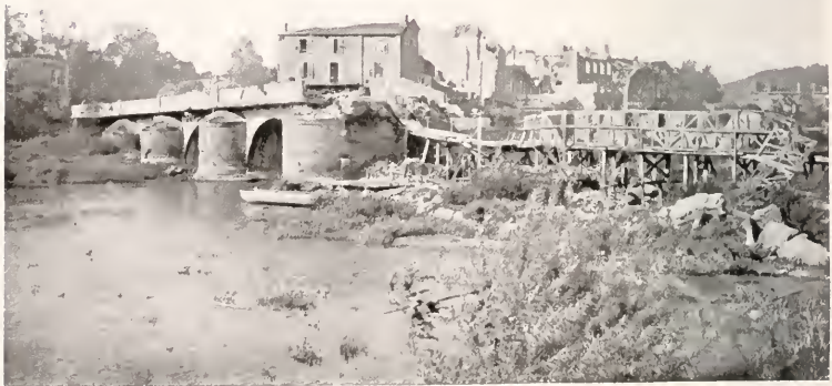
DESTROYED BRIDGE OVER THE MEUSE
