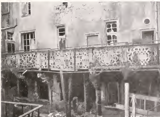
OLD RENAISSANCE BALCONY AT NO. 7, RUE ST. LAURENT
