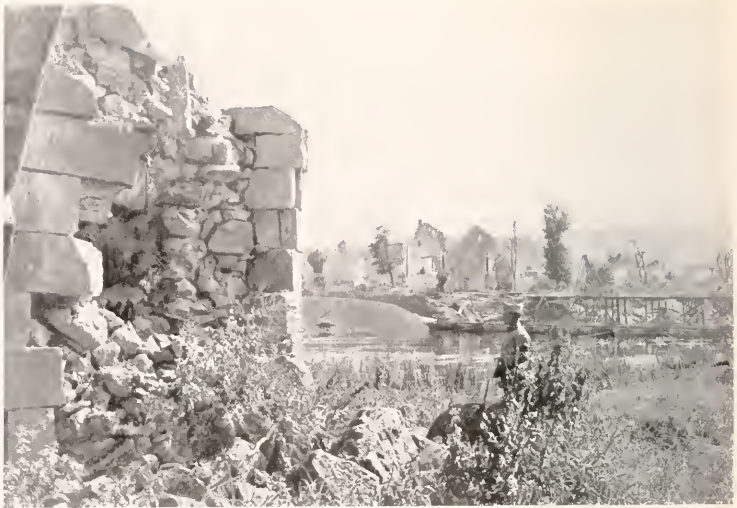
THE DESTROYED BRIDGE AT ST. MIHIEL
