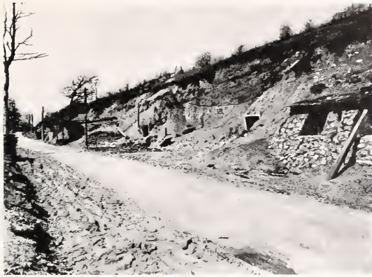
ROAD FROM CALONNE TRENCH TO ST. REMY German shelters and dug-outs.
