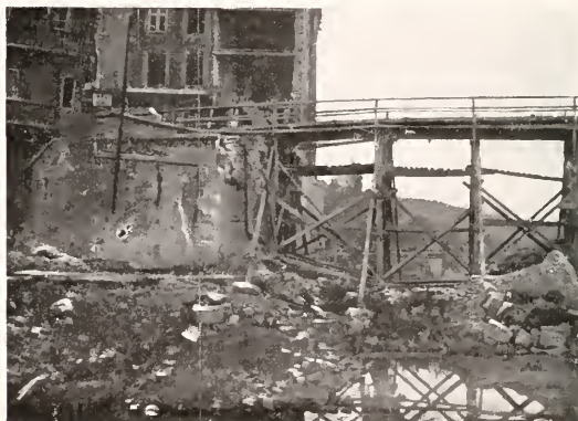
TEMPORARY BRIDGE OVER THE MOSELLE (left bank)
