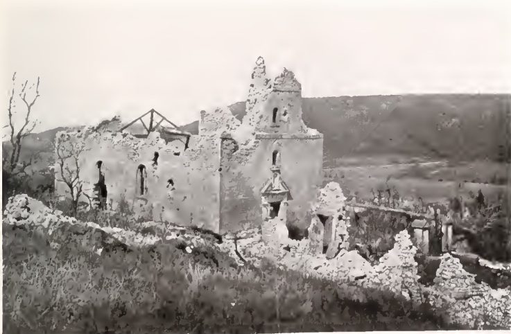
RUINED CHURCH AND VILLAGE OF ST. REMY In the background: Combres Crest (right), Eparges Crest (left).
