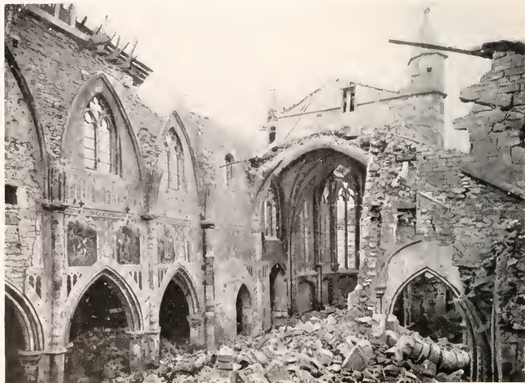
ETAIN CHURCH. CENTRAL NAVE SEEN FROM THE CHOIR
