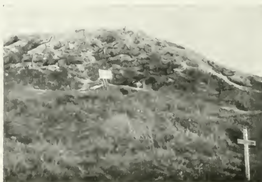
ENTRANCE TO THE UNDERGROUND DEFENCES.
