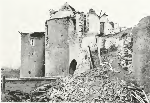
PÉRONNE. THE FAÇADE OF THE CHÂTEAU AT THE END OF THE WAR.
