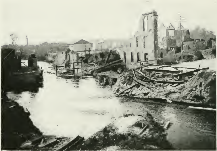
THE DESTROYED BRIDGE ON THE OLD RAMPARTS. On the right is the end of the Rue St. Fursy.
