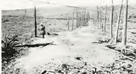
THE SITE OF MONACU FARM ON THE MAUREPAS ROAD NEAR HEM WOOD.
