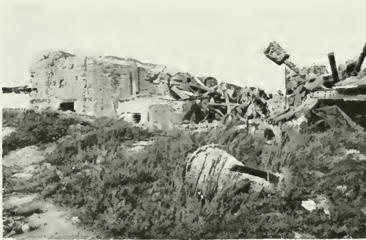
GERMAN OBSERVATION-POST OF CONCRETE, IN THE ENGINE-ROOM.
