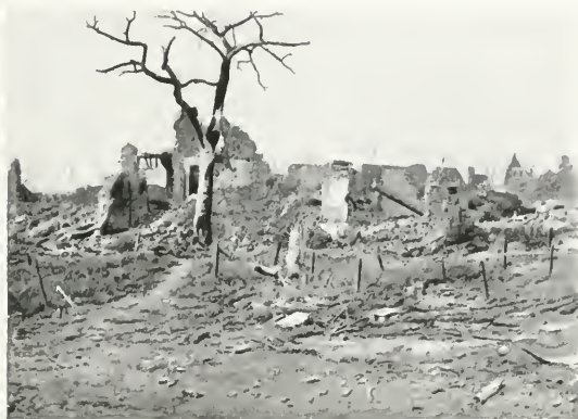
MONT-ST.- QUENTIN. RUINED HOUSES.
