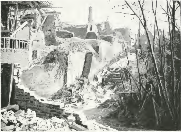
RUINED WORKS ON RIVER ANCRE, AND CASCADE.
