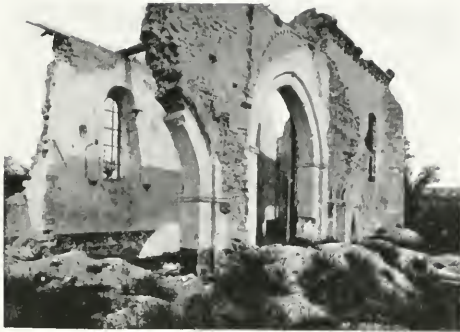
CURLU CHURCH. Fragment of 13th century wall—all that is left of the village.
