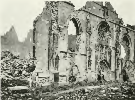
THE FAÇADE OF ST. JEAN CHURCH IN 1919.
