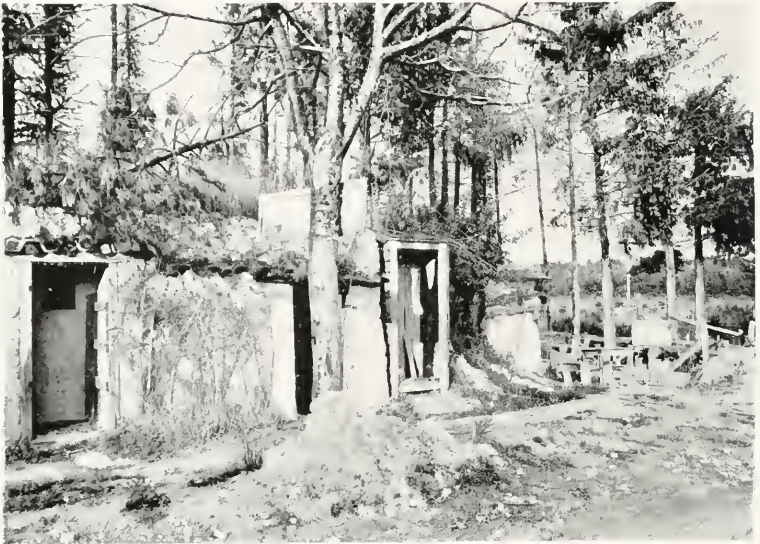
FRENCH DEFENCE WORKS BETWEEN SERVON AND ST. THOMAS
