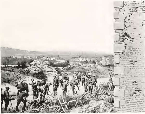
BOUREUILLES. D. CO. OF 11TH ENGINEERS ROAD-MAKING
