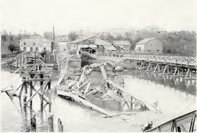
MOURON. DESTROYED BRIDGE OVER THE AISNE, AND TEMPORARY BRIDGE
