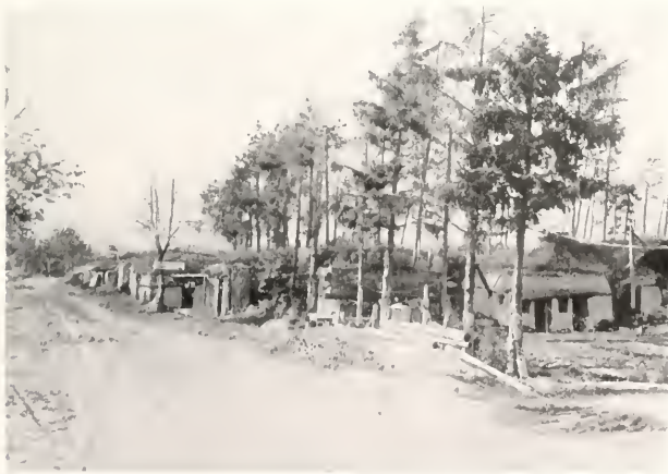
FRENCH DEFENCE WORKS AND DRESSING-STATION G.C. 66, between Servon and St. Thomas.
