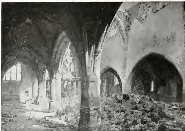
CLERMONT- EN- ARGONNE. CHURCH NAVE, SEEN FROM NORTH AISLES
