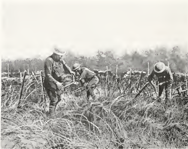
CHEPPY. DETACHMENT OF 107TH ENGINEERS (32ND INF. DIV.) CLEARING ROAD OF BARBED-WIRE ENTANGLEMENTS
