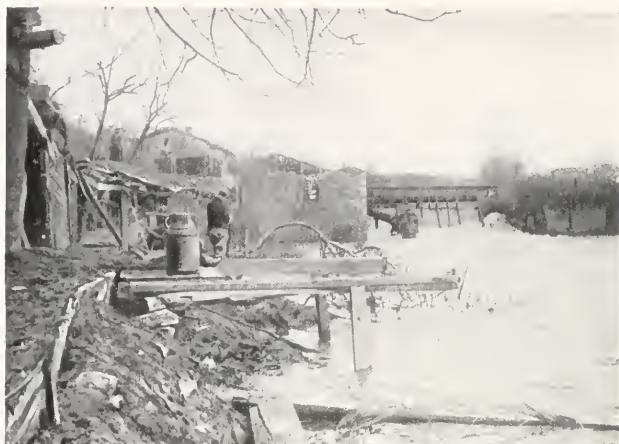
NEUVILLY. RUINS OF ELECTRIC POWER STATION ON RIVER AIRE
