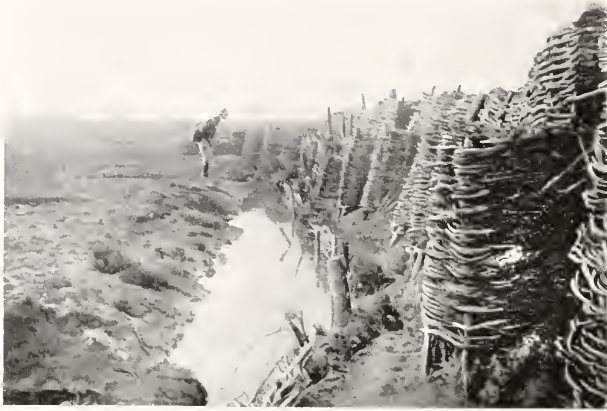
FIRST FRENCH LINE IN AISNE VALLEY, BEFORE SERVON ( St. Thomas' Sector. )
