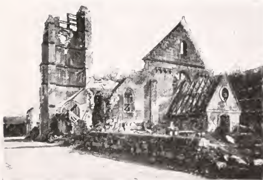
RUINED CHURCH OF ST. BANDRY.
