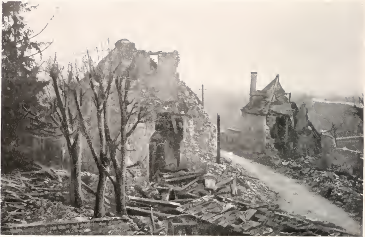
RUINED CHURCH AT MONT-ST.-PÈRE.
