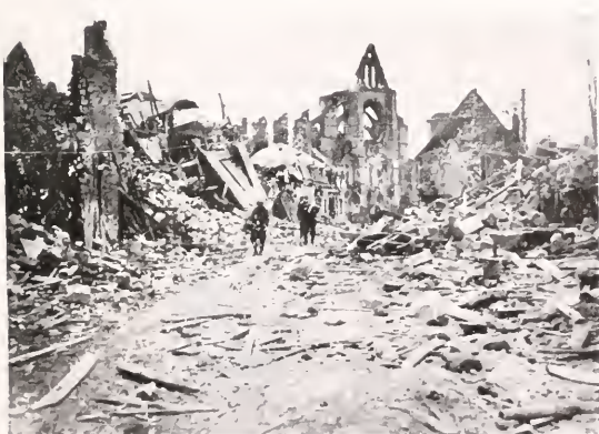
LONGPONT ABBEY CHURCH, SEEN FROM THE STREET LEADING TO THE FORTIFIED GATE.
