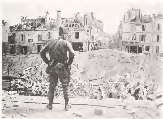
CHÂTEAU-THIERRY BRIDGE AFTER IT WAS BLOWN UP.
