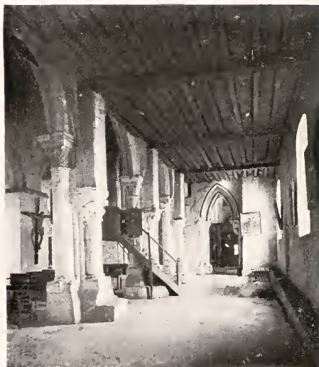
INTERIOR OF GLENNES CHURCH.
