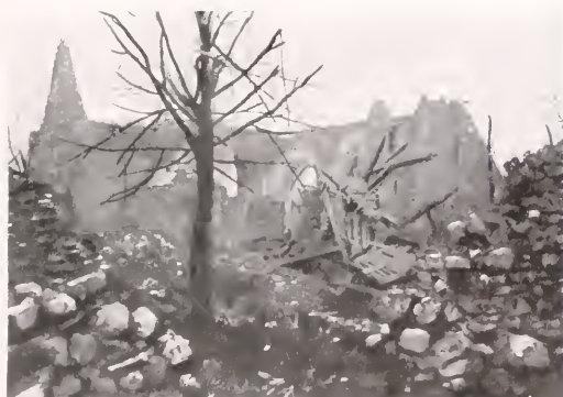
DOMMIERS CHURCH IN RUINS.
