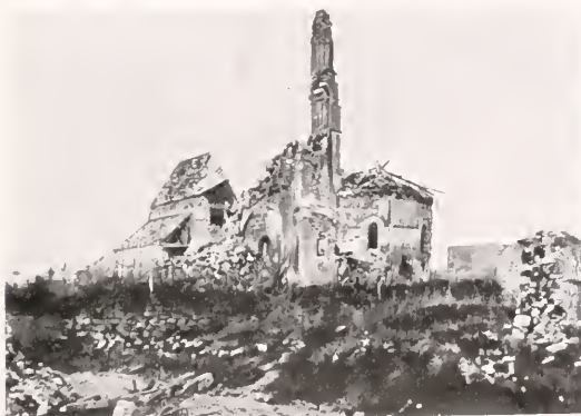
RUINED CHURCH OF OULCHY-LA-VILLE.
