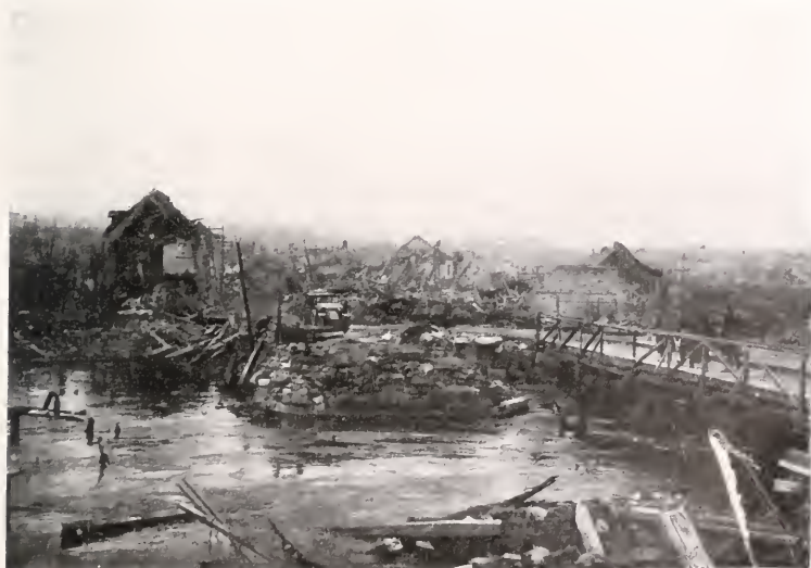
RUINS OF FISMES SEEN FROM THE TEMPORARY BRIDGE OVER THE VESLE WHICH CONNECTS THAT VILLAGE UP WITH FISMETTES.
