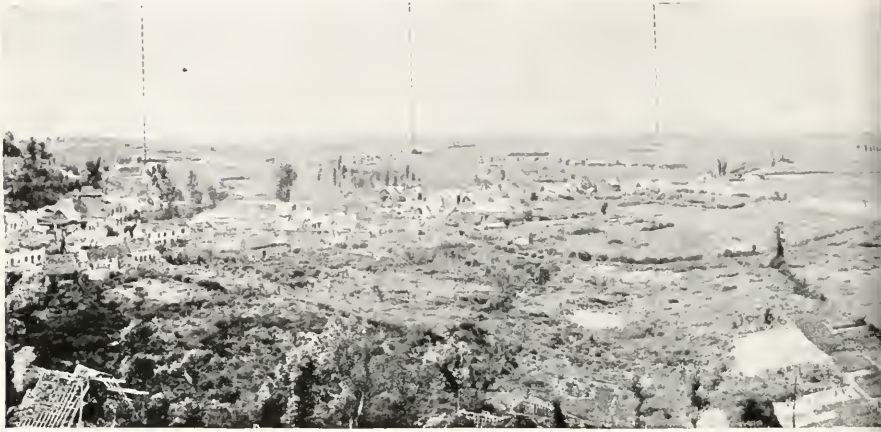
PANORAMIC VIEW TO THE WEST AND SOUTH OF MONTDIDIER
