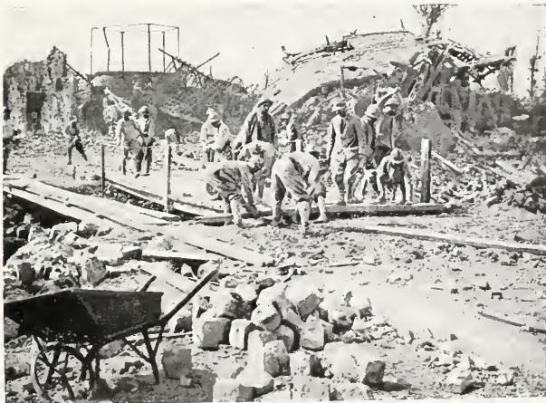
MONTDIDIER. BUILDING A BRIDGE IN FRONT OF THE STATION.
