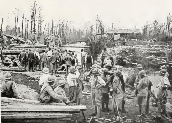
BUILDING A BRIDGE ACROSS THE AVRE, NEAR MOREUIL.
