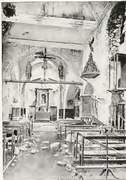
MARGNY-SUR-MATZ. — INTERIOR OF THE CHURCH. Note the "Glory Beam".
