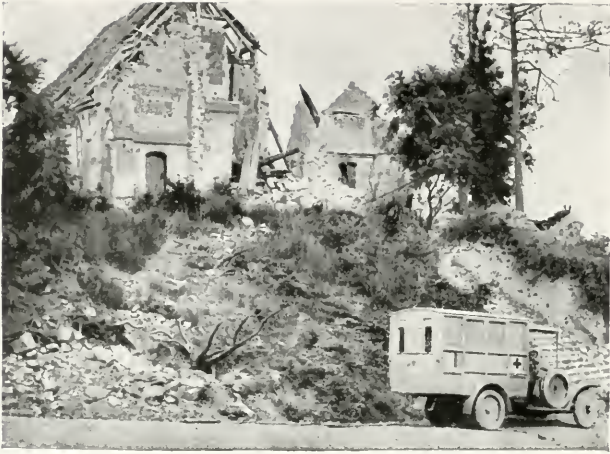
BOULOGNE-LA-GRASSE. — THE RUINED CHURCH.
